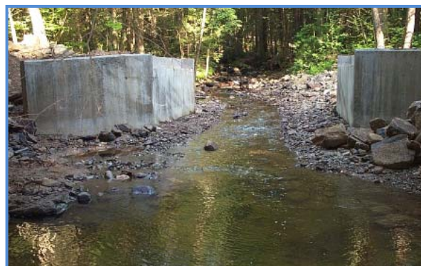
Culverts were removed in 2011, providing upstream fish passage. This site is being readied for bridge installation.
