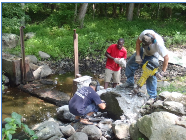
TNC and DEEP staff at work removing one of the two concrete dams on the Aspetuck River in Weston.
