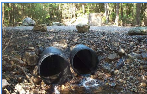
Perched culverts (2006) that blocked upstream fish passage.
